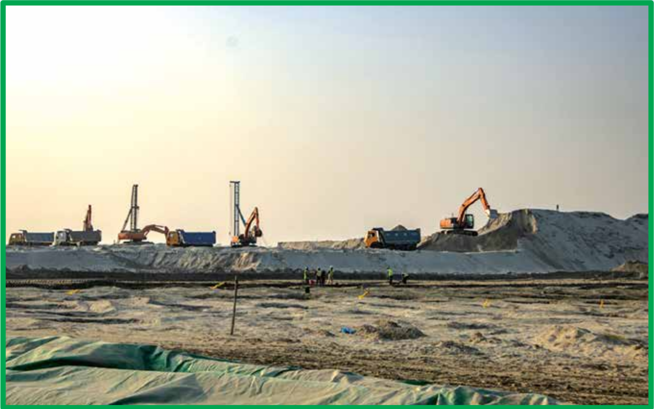
Soil Improvement of Coal Yard Area
