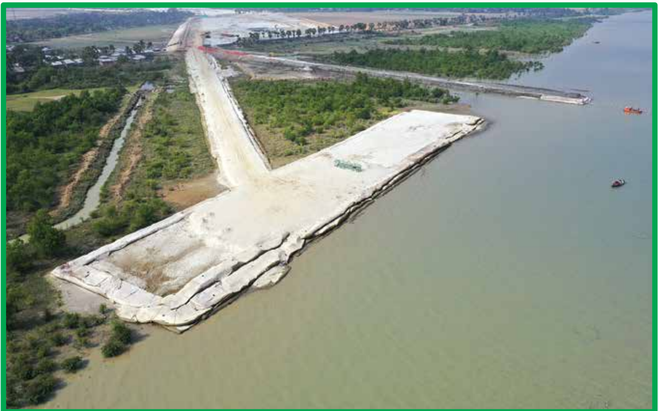
Under Construction Jetty at Project Site
