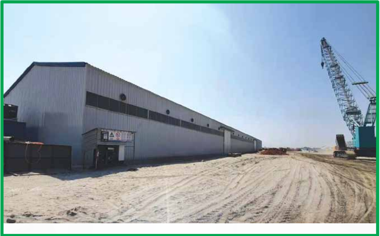
Warehouse Building at Project Site
