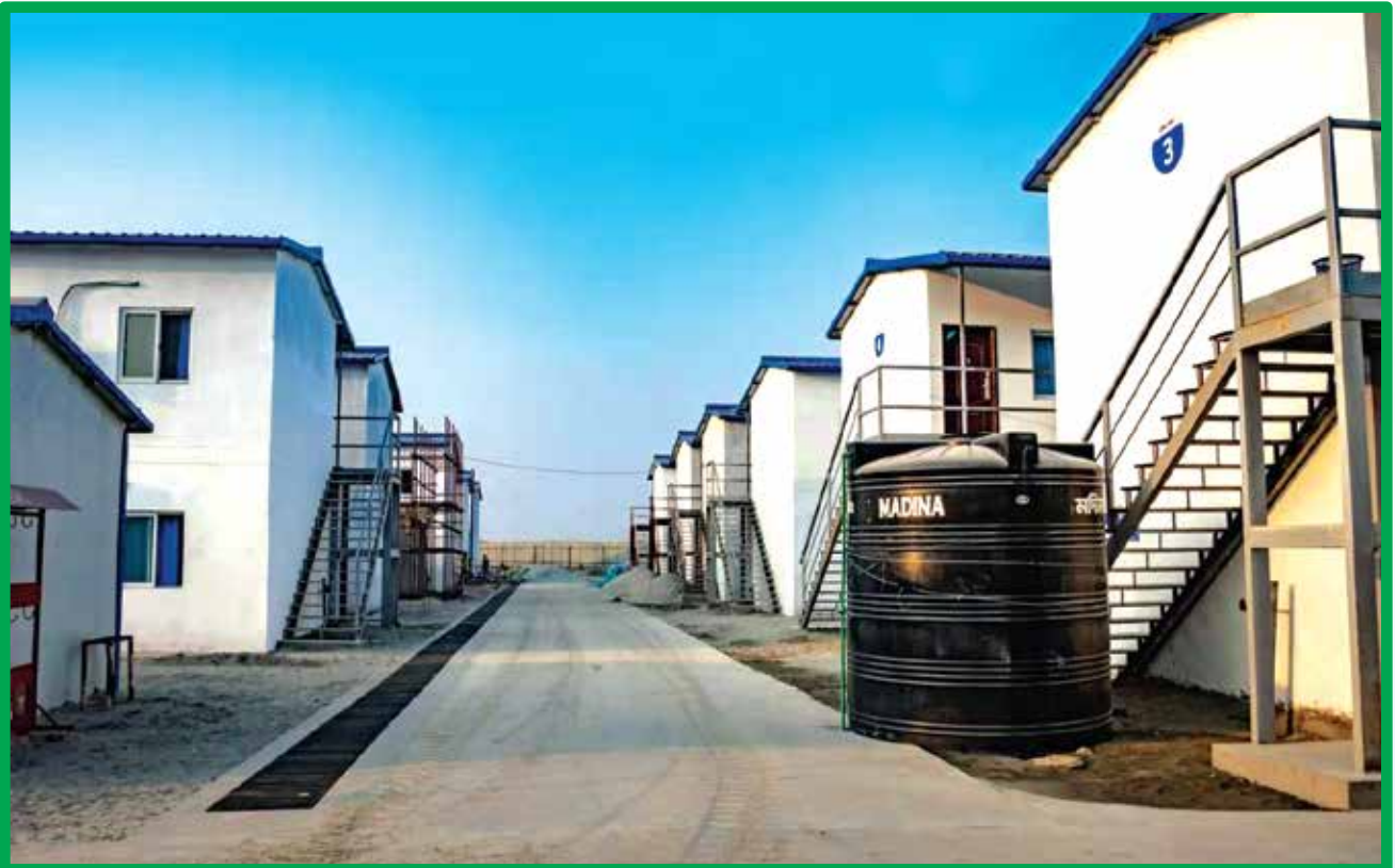
Chinese Personnel Dormitory at Project Site
