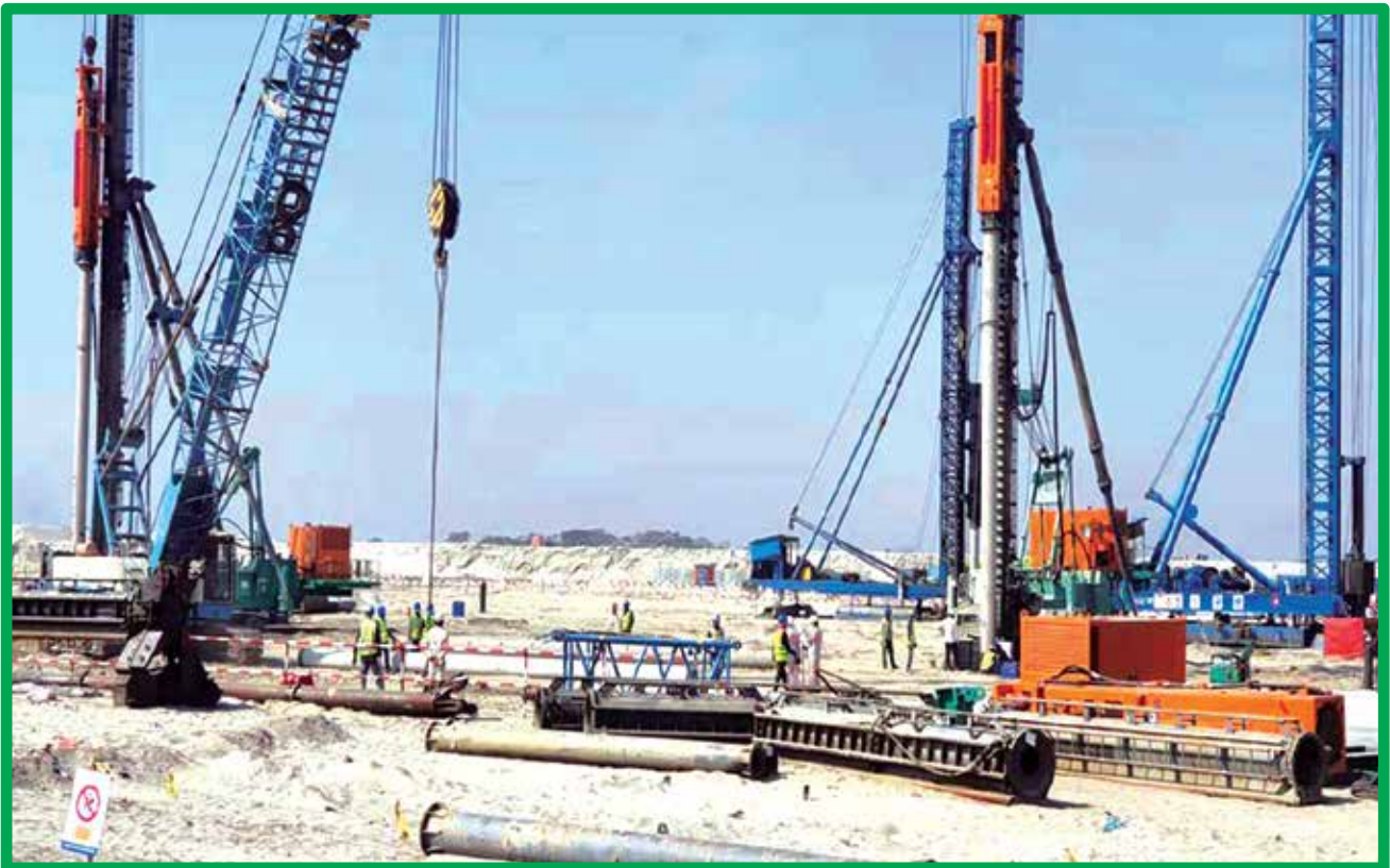
Pilling Works at Project Site
