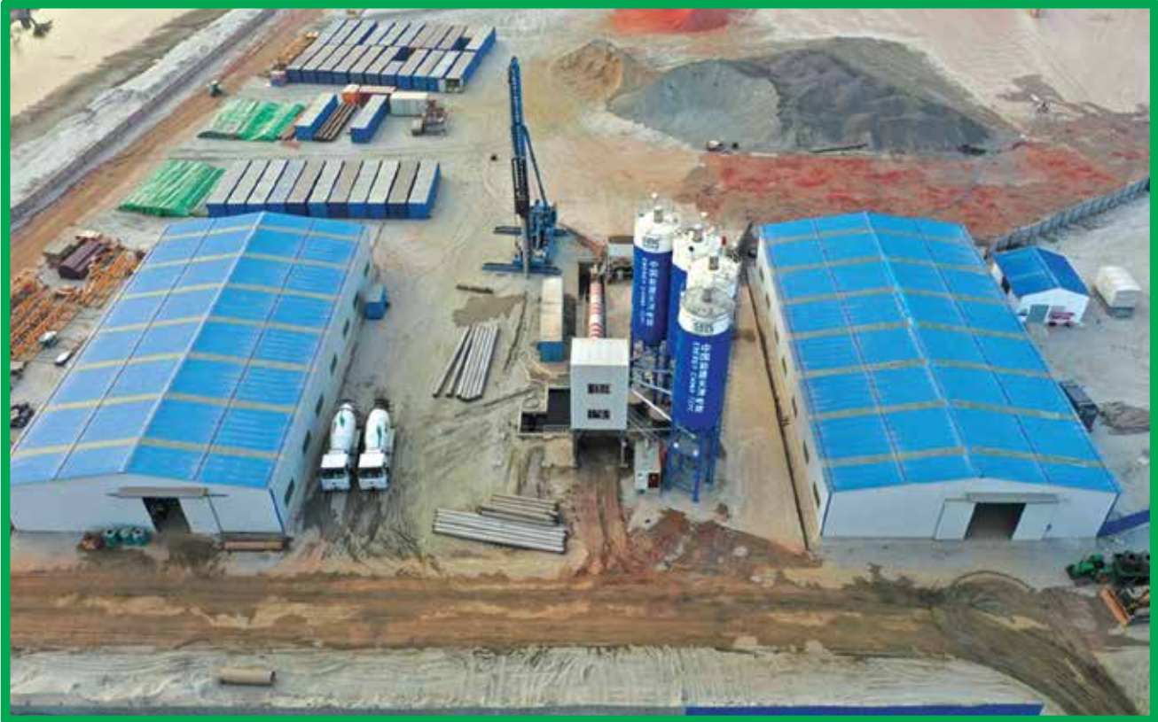
Batching Plant at Project Site
