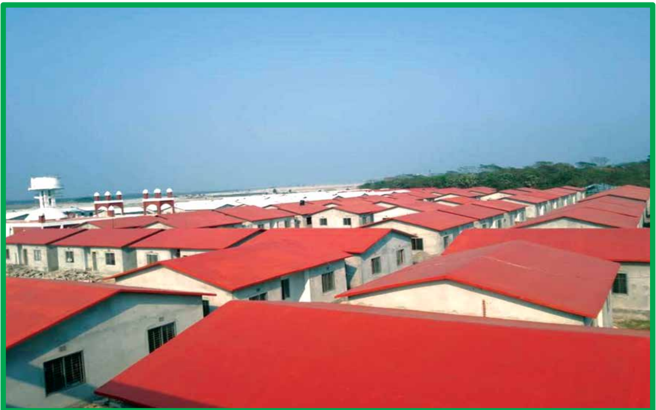
Houses at Resettlement Area
