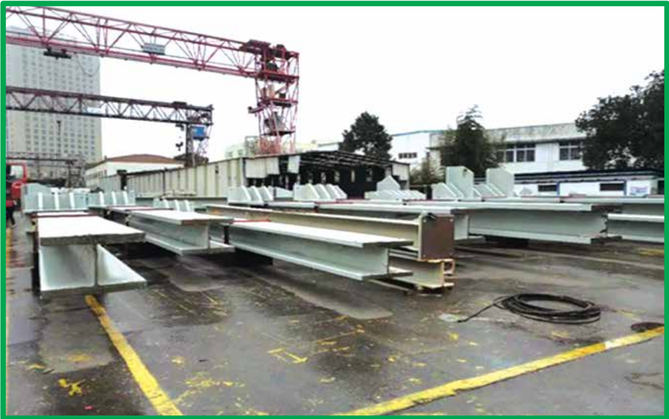
Steel Structure Boiler No # 1 Manufacturing at Factory, China
