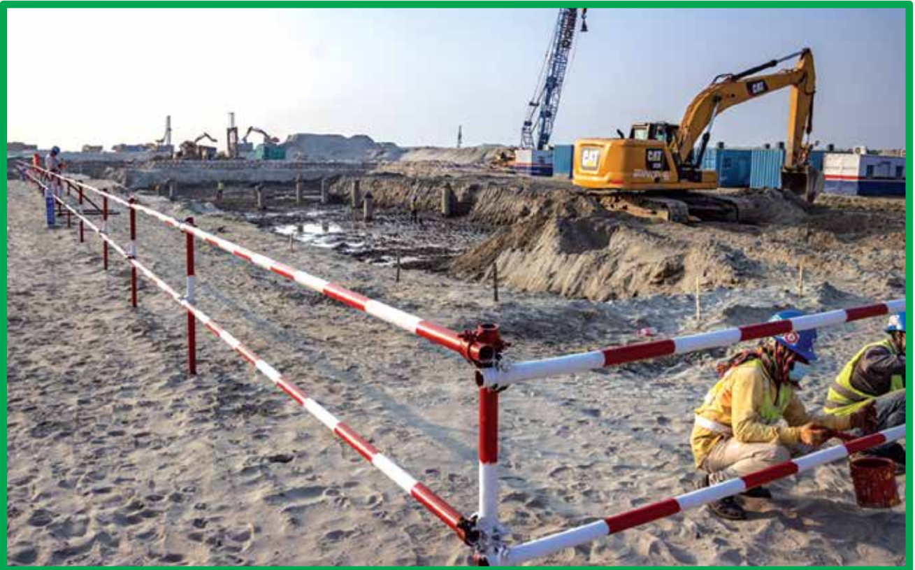
Construction Works at Project Site
