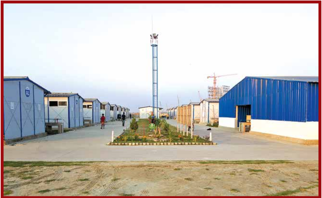
Temporary Living Dormitory for workers
