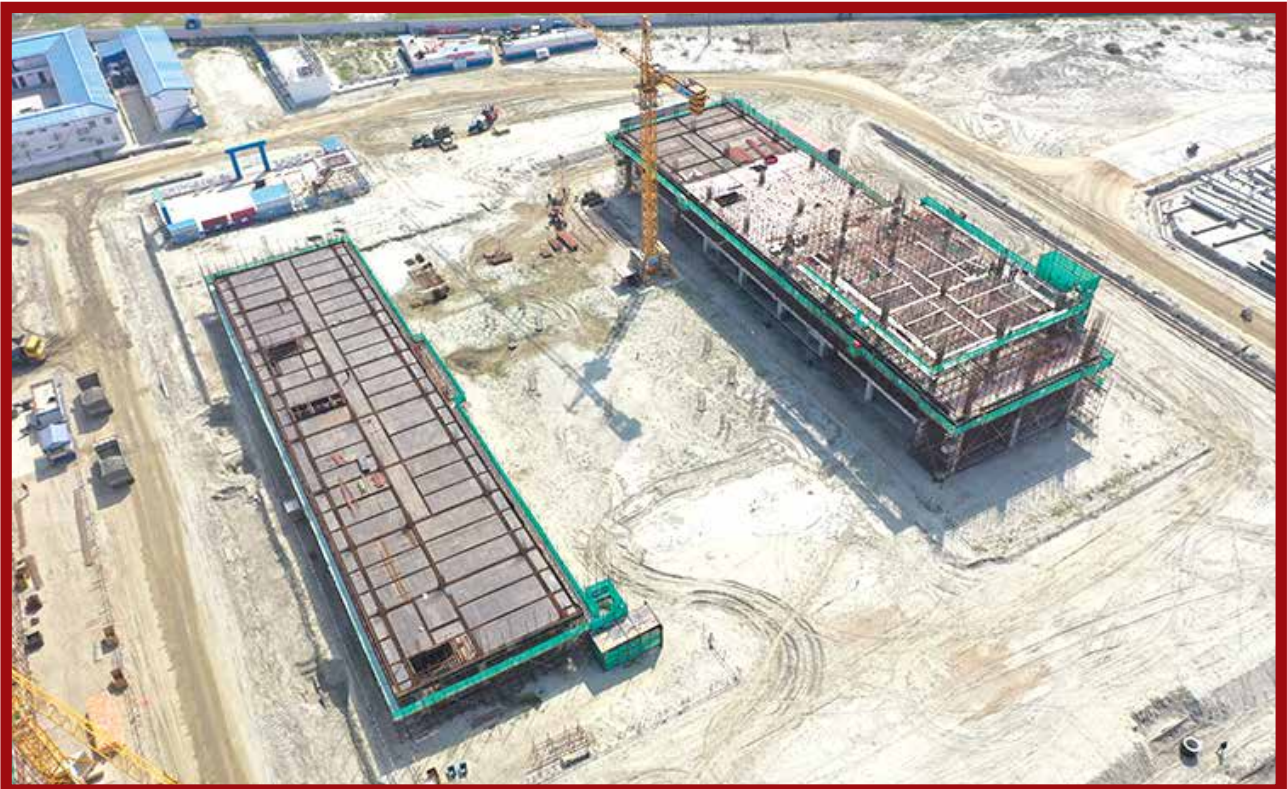
Admin & Engineering Building
