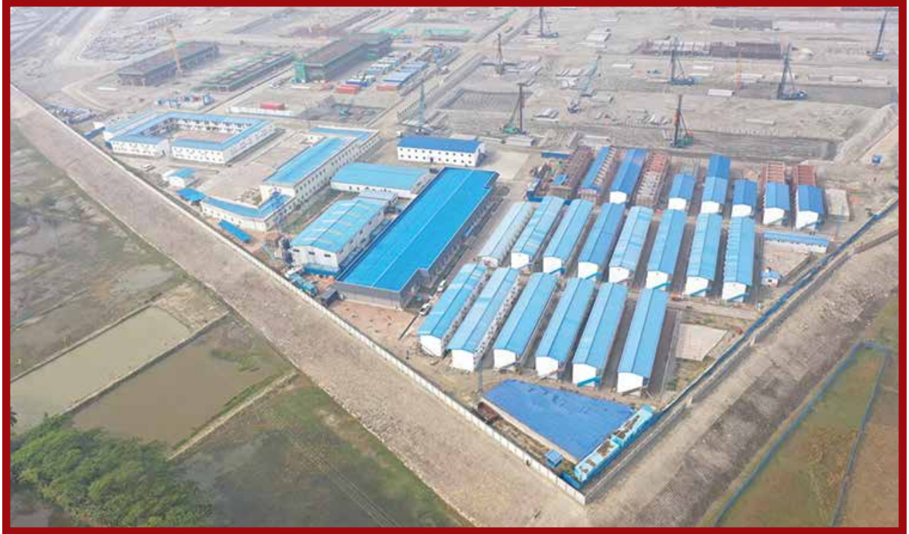
Temporary Living Dormitory
