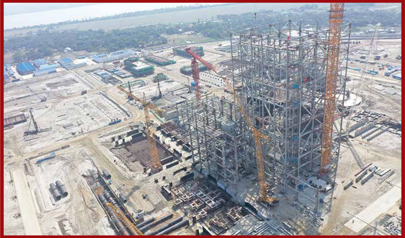
Boiler Super Structure
