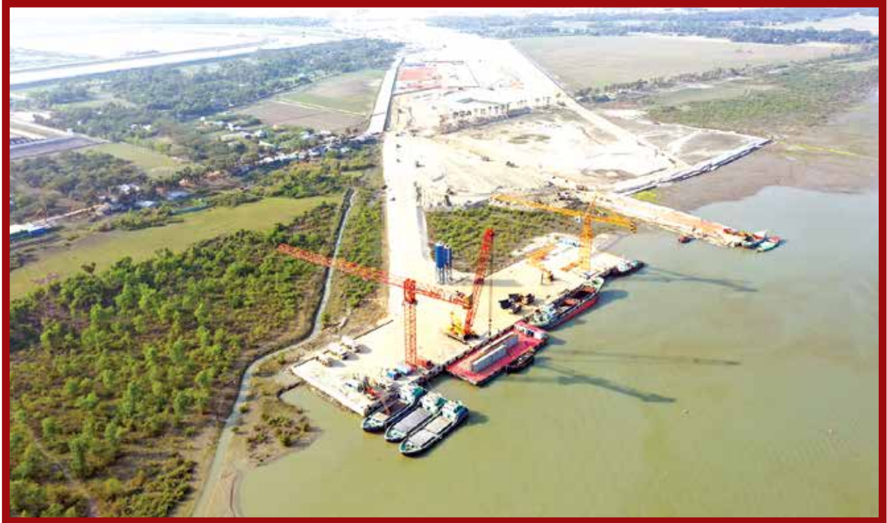
Material Handling Jetty
