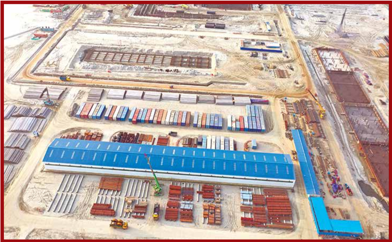
400 KV GIS Sub-Station Yard
