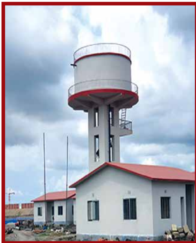
Water Supply Facility
